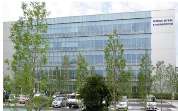
Kitakyushu Technology Center of Nippon Steel Engineering
